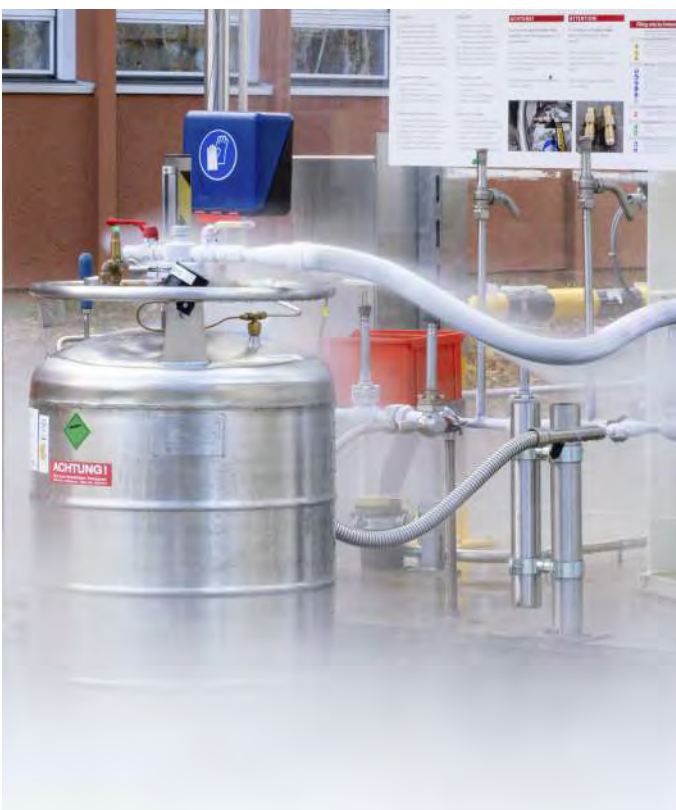
Filling of a DEWAR with liquid nitrogen
