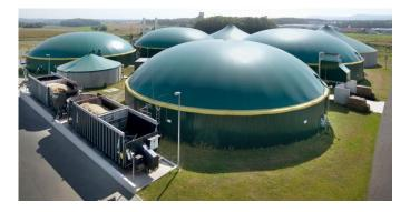
**Biogas plant.** Organic waste and grease separator content are collected on fixed intervals by a suction truck and then taken to the biogas plant where thy are treated at 70°C in a bio digester. After an anaerobic process, 1 m³ of organic waste turns into 140 m³ of biogas. Biogas is a mixture of methane and carbon dioxide, the first of which can be combusted to produce green renewable energy. The residues after digestion are used in agriculture as fertiliser and soil conditioner.
