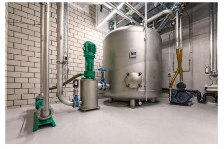
Collection central. The kitchen bio waste is collected, crushed and stored in a hermetically closed tank. No odours arise inside the building due to the permanently vacuum in the pipe system. The filtered exhaled air is routed over the roof. The plant technology is operated with a SPS central control system. The inlet stations are connected to the central control system via a bus system. The operation is fully automated.
